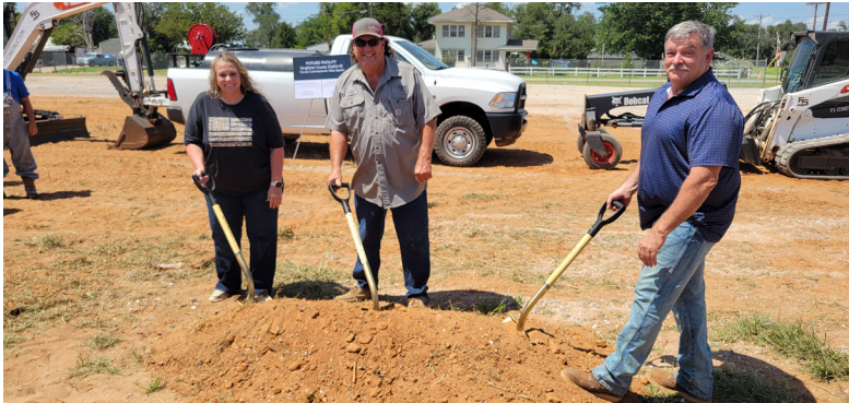
Pictured are Alisha Haymaker, Clay Vincent, and Mike Sparks breaking ground for the new county building.
