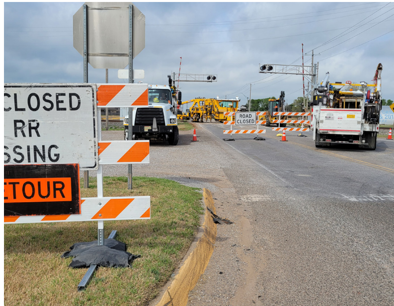
Railroad crossing repair at US Highway 51 photo by AAH Jack Quirk
