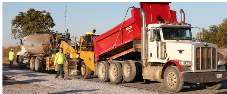
Chip-and-seal crew lays down the first layer of two that will complete the new road surface.
